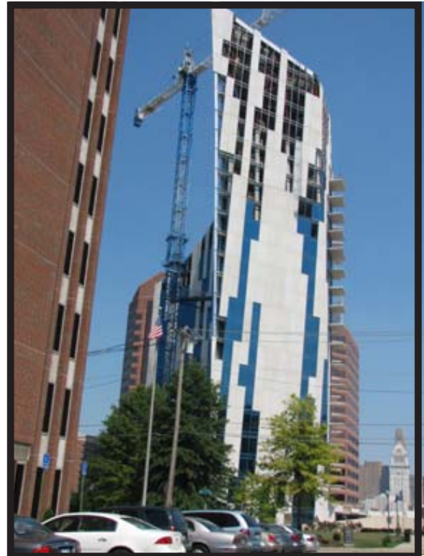
Construction continues at The Ascent at Robling Bridge in Covington, KY.
